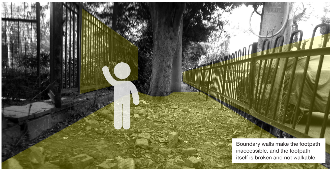
Figure 1.16 Inaccessible walking zone (Panchsheel Park South, New Delhi)
